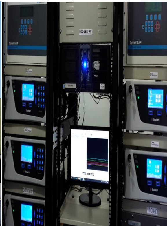
2.2 – Inside view of Station
