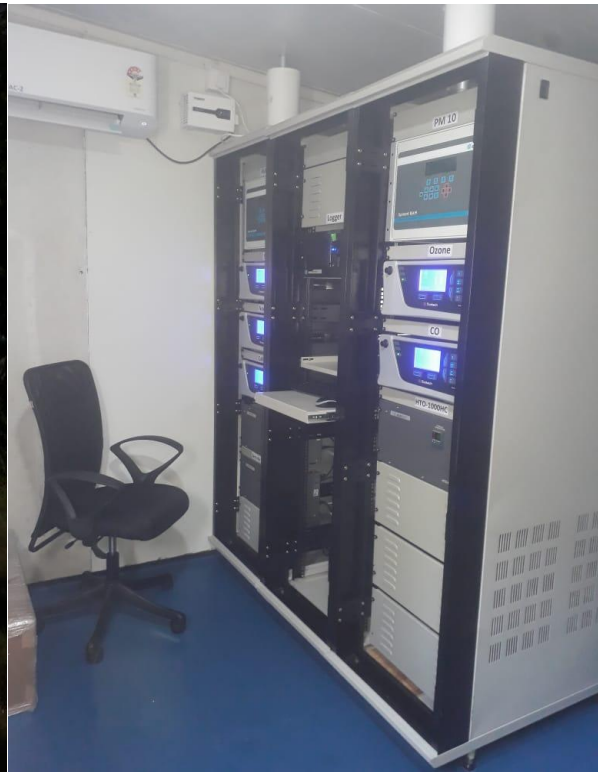
1.2 - Inside view of Station
