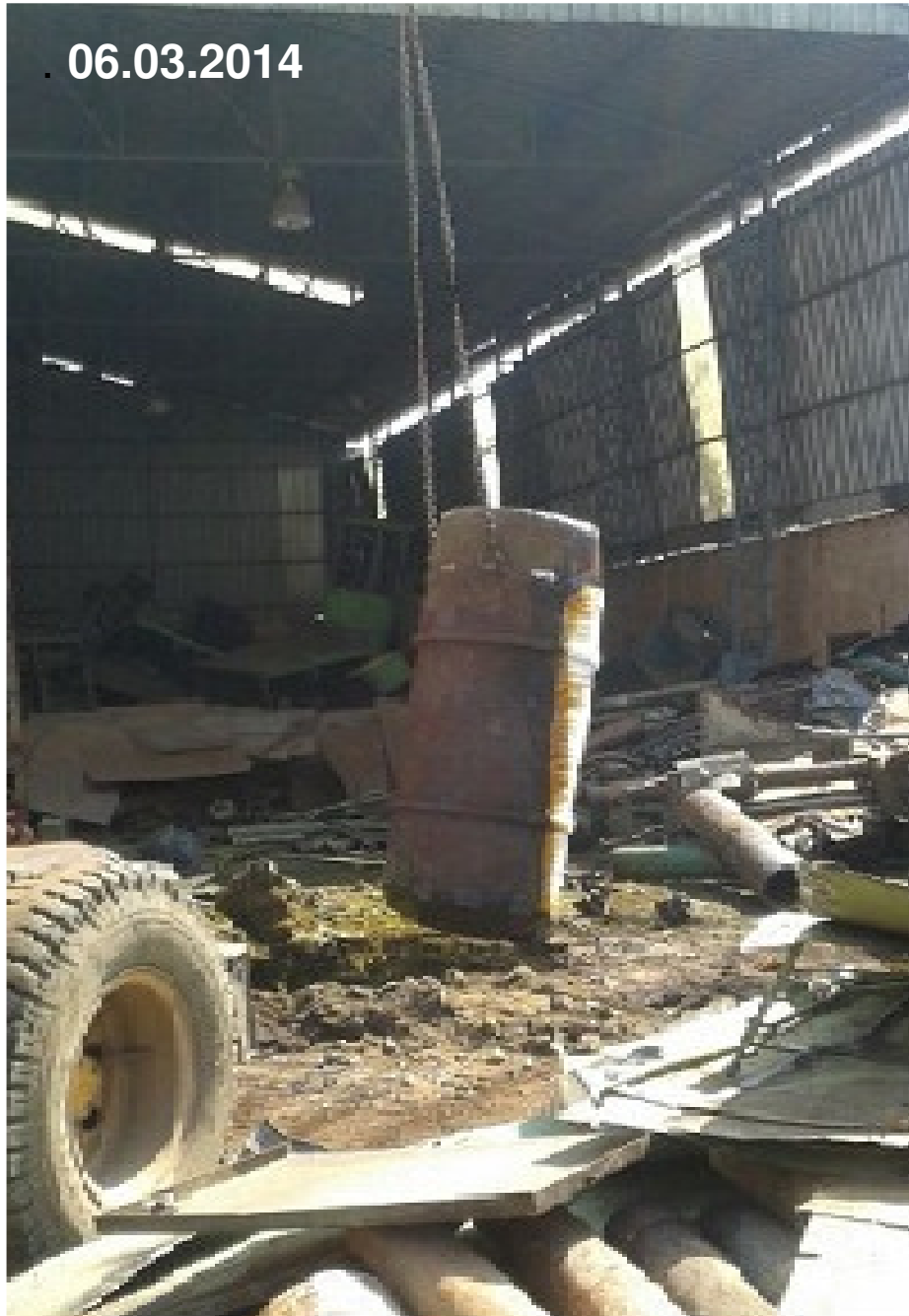
The Cylinder being lifted & lowered in to the temporary Pit
