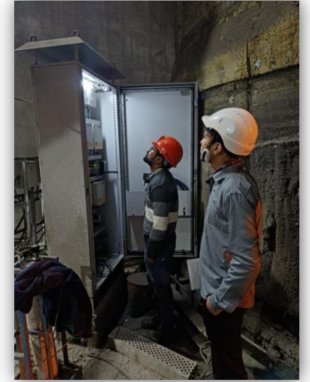
Pre deployment inspection
