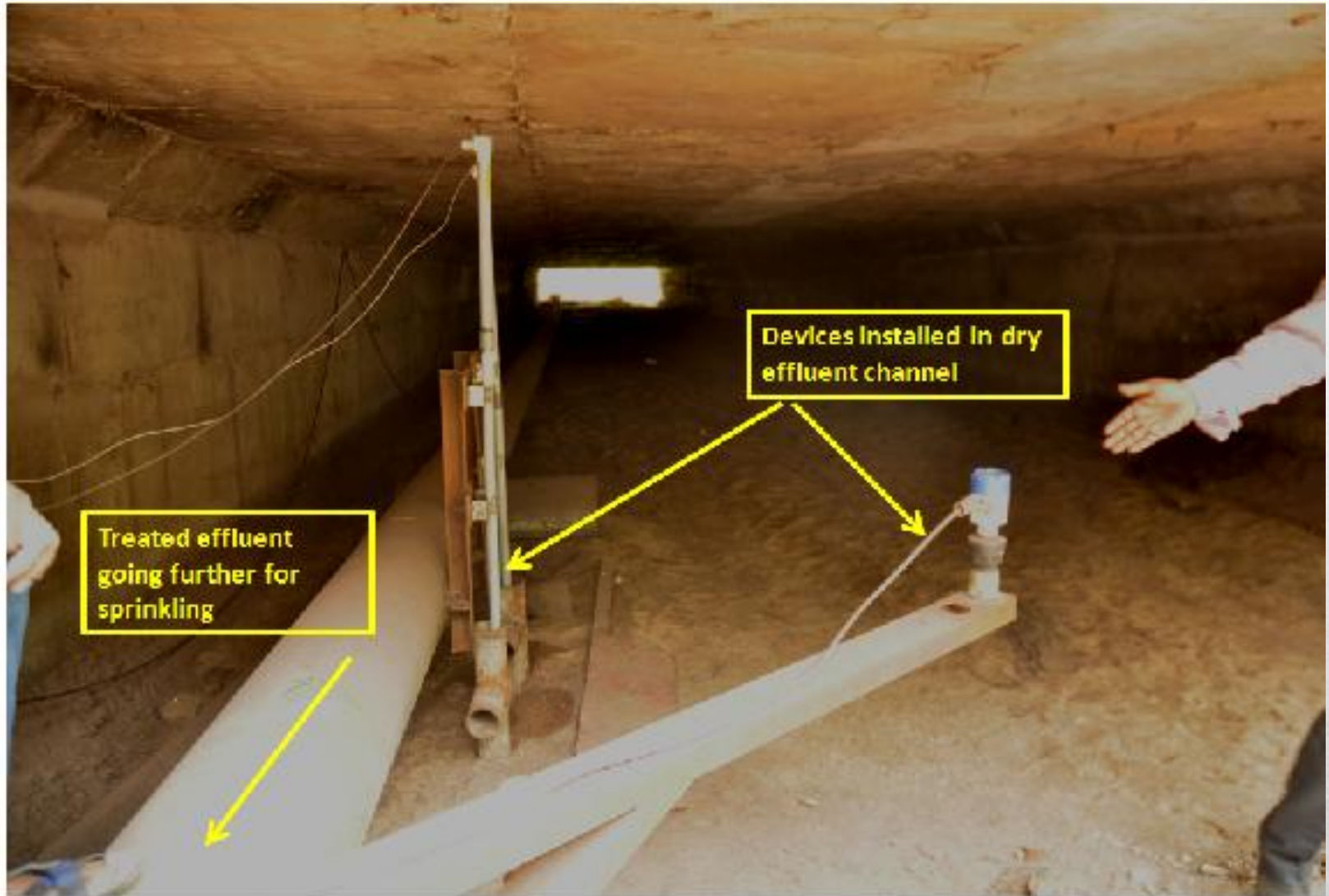
CSE's survey: installation of CEMS
