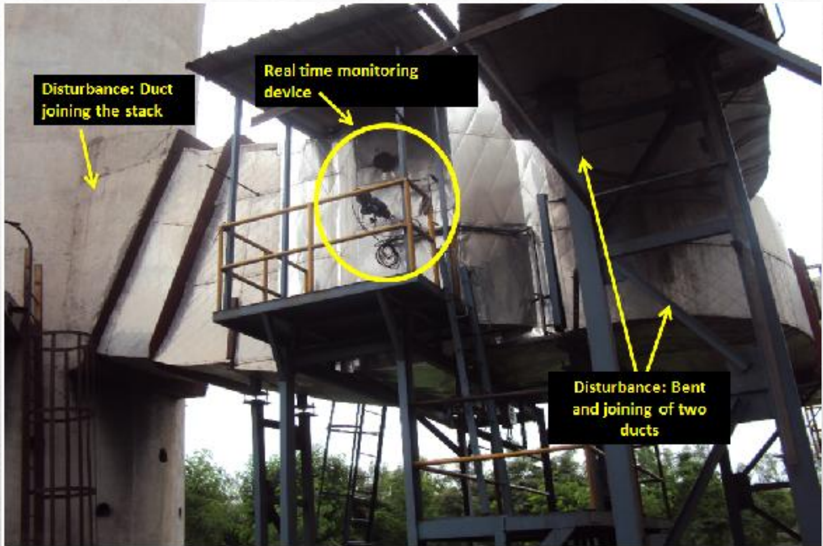
CSE's survey: installation of CEMS
