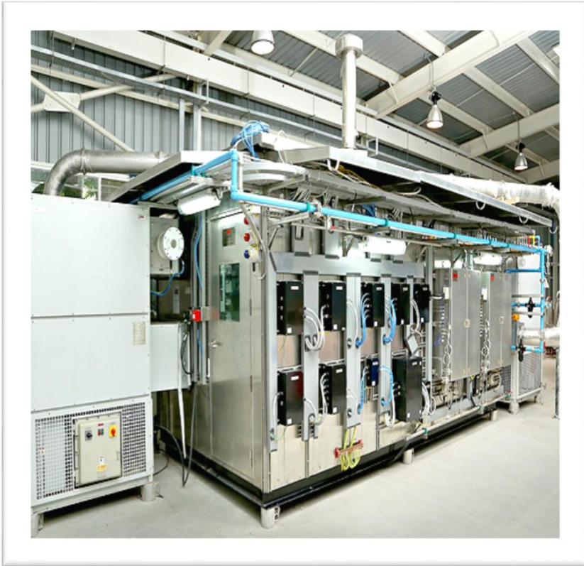
Emission Systems in Shelters
