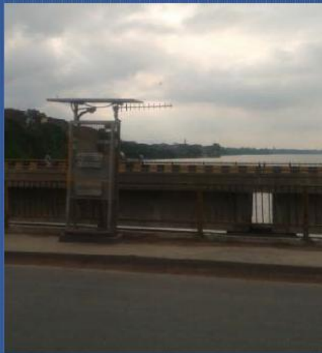
Vertical Bridge Spanning
