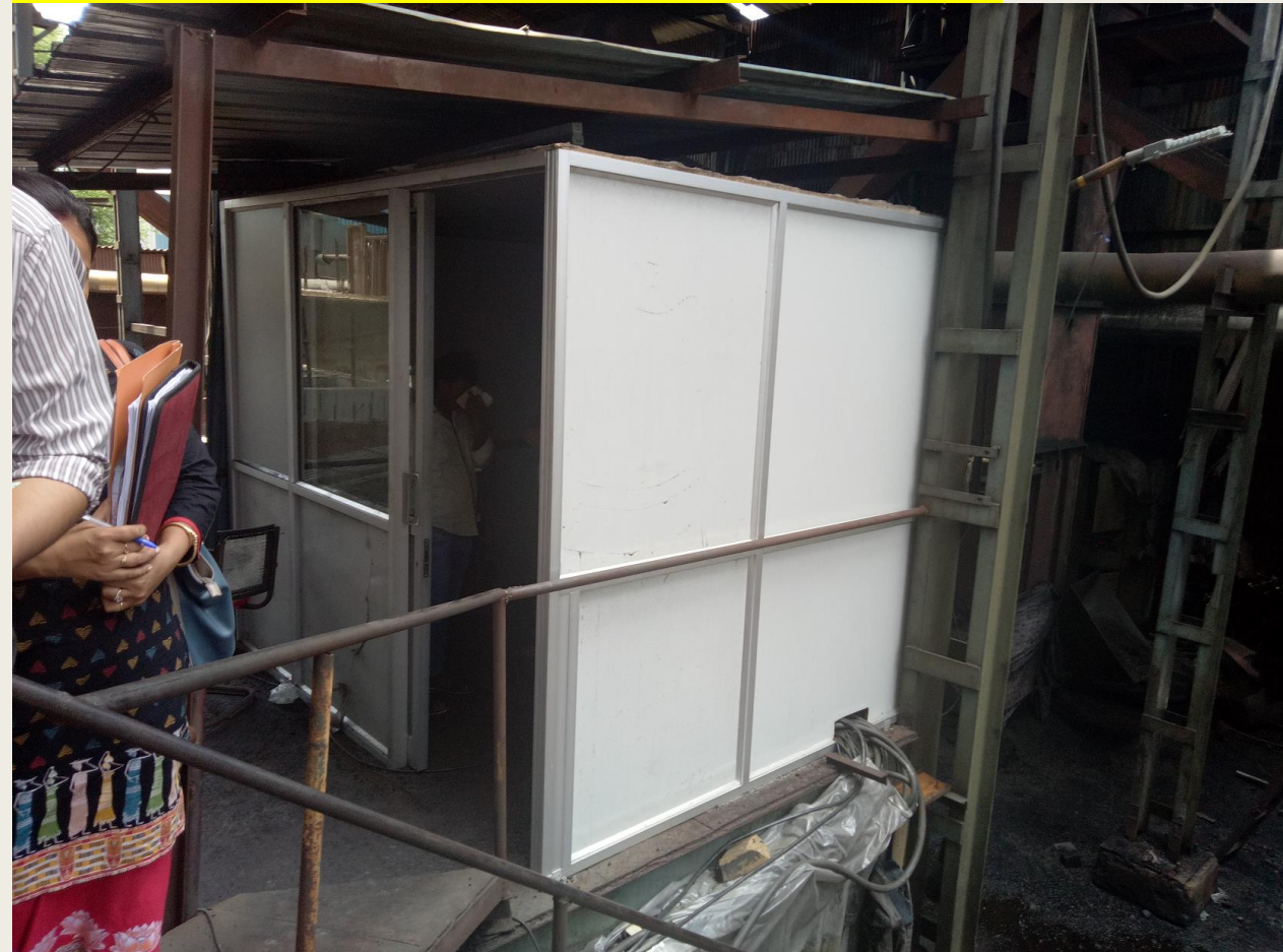
CEMS cabinet with no AC, Fan, Light
